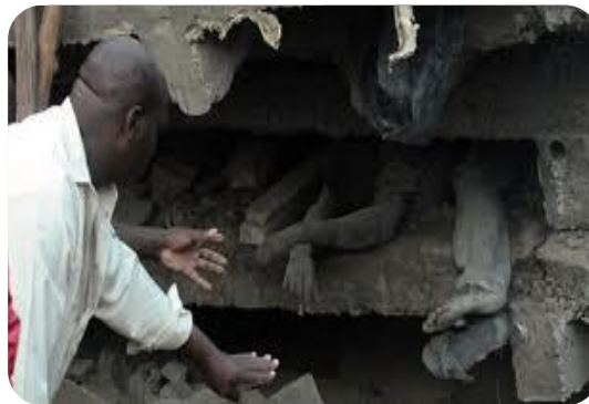
Fig 3: Trapped workers in a collapsed 4-storey building.
