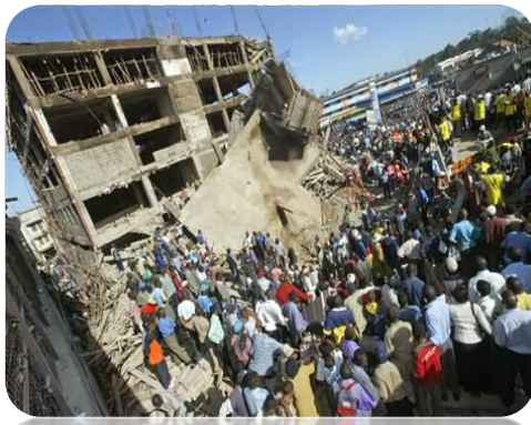
Fig 2: collapsed five storey building in Nairobi
