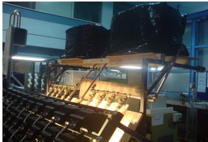
Fig. 3. Insulated water tanks and artificial insulation
