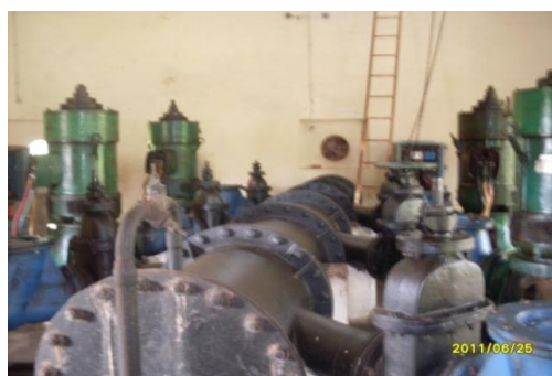
Figure 3:- Pump House at Lalpur (Jabalpur) water treatment plant
