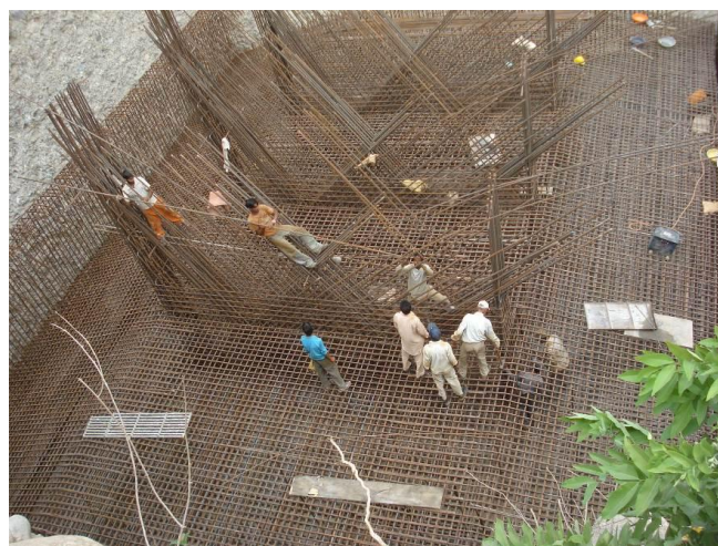
Photo 5: Reinforcement cage for foundation, arch ribs & piers (Baner khad bridge)
