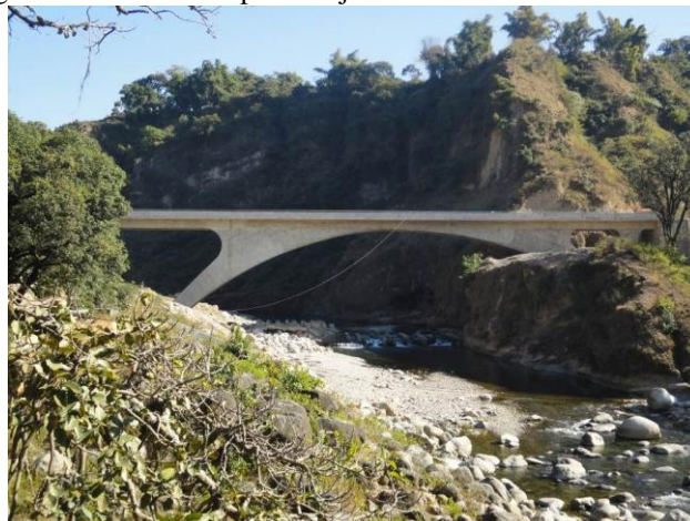
Photo 1: Baner khad bridge on NH88 (Himachal Pradesh)
