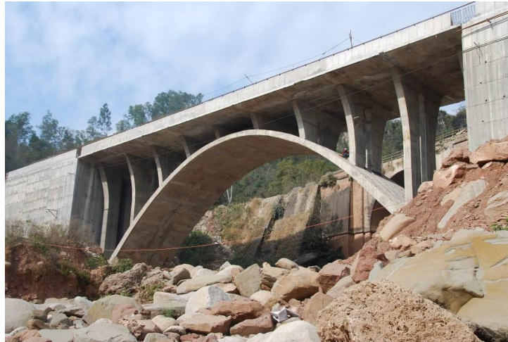
Photo 3: Trilokpur bridge on NH20 (Himachal Pradesh)
