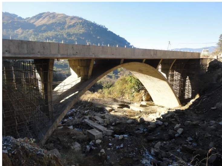
Photo 4: Nagrota nallah bridge on NH20 (Himachal Pradesh)
