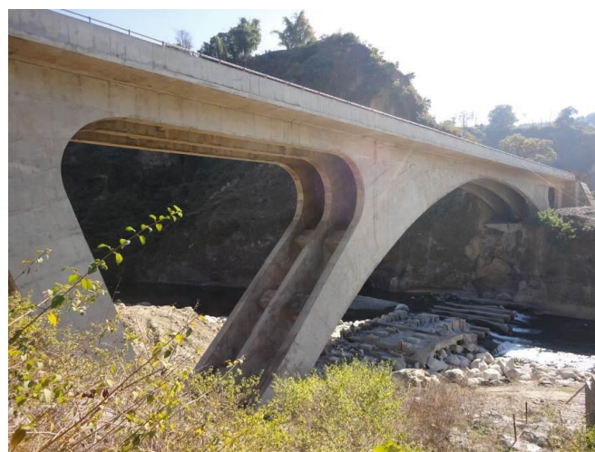
Photo 2: Baner khad bridge on NH88 (Himachal Pradesh)
