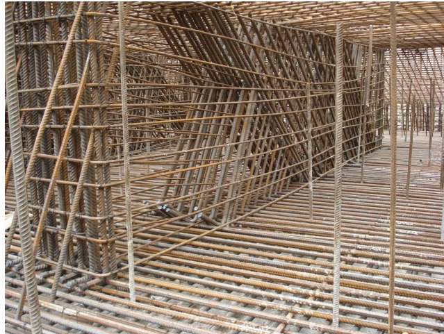
Photo 6: Reinforcement cage for foundation, arch ribs & piers (Baner khad bridge)
