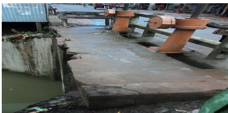
Picture 8: Sluice gate for controlling the saline water intrusion.
