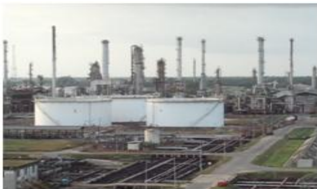
Photograph 3.2: Storage Tanks and Plant Towers in a Refinery. (Source: wwpennpcng, June, 2013).
