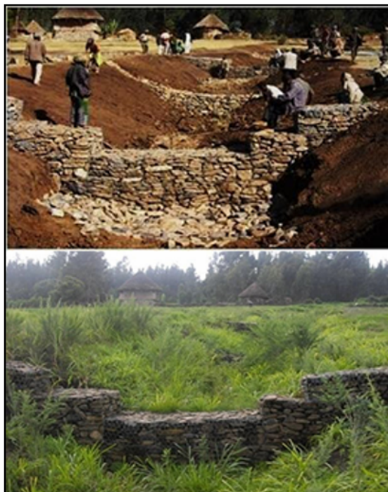
Figure 8: Soil and Water Conservation efforts (Source; Blue Nile Water Resource Authority)
