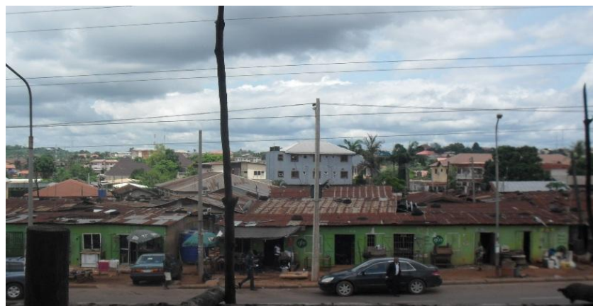
Plate 9. Upper Chima Avenue, New Haven, Enugu slum Source: Obiadi (May, 2016)
