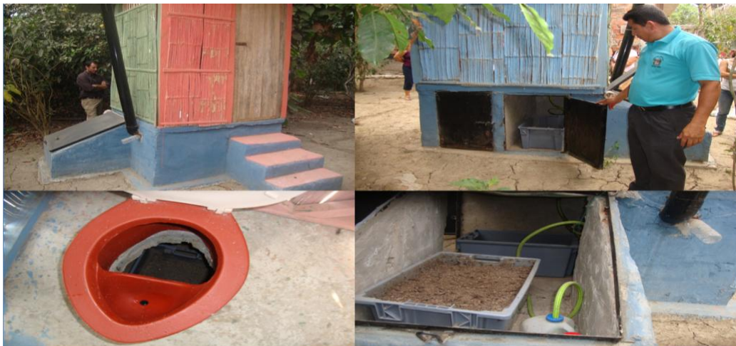
Image 1. Sanitation unit built up under a PCP approach in Junín, Ecuador. Photo: Bruno Bellettini
