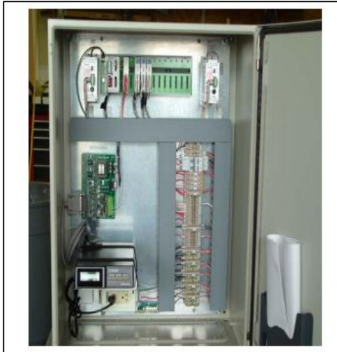
Fig. 3 (a) RTU configured with PAC Fig. 3(b) Control Panel
