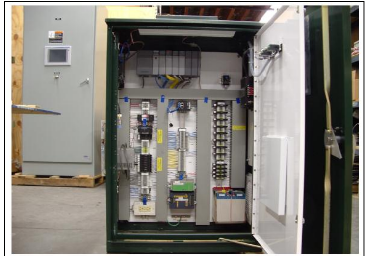
Fig. 3 (a) RTU configured with PAC Fig. 3(b) Control Panel
