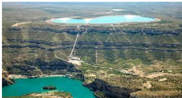
Figure. 3 shows Artificial lake on river side
