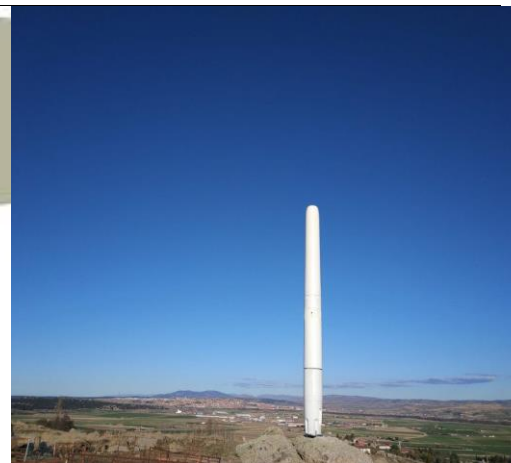
Figure. 8 shows vertical wind turbine
