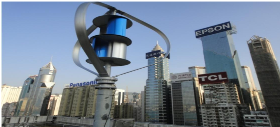
Figure 2.3.2. - Vertical axis wind turbines (VAWT) on the commercial building
