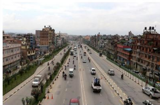
Figure 3: B&B Hospital (Section 2)
