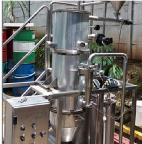
Fig 1. Concurrent flow gasification reactor.
