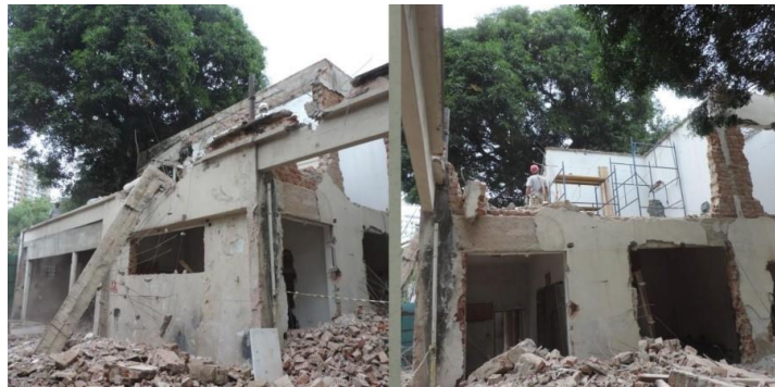
Figure 7: Structural System Elements Of Block F (In The Process Of Demolition) 17 .
