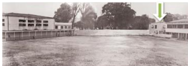
Figure 4: View Of The Completed Original Block F (Indicated By The Arrow) 14 .
