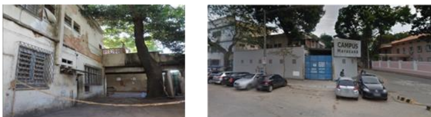
Figure 6: Side View Of Block F And Partial Rear View, Respectively 17,18 .
