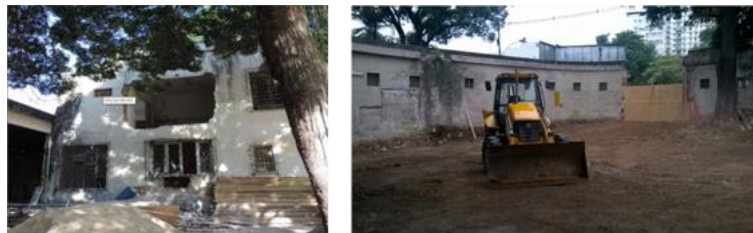
Figure 8: Demolition Of Block F: Beginning And End 17 .
