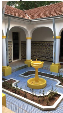
Figure 13 - Detail of the internal garden of the House of Luiz de Souza Leão.
