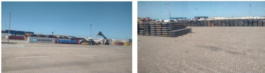
Figure 1: Container Yard and Steel Plates at the Port of Pecém
