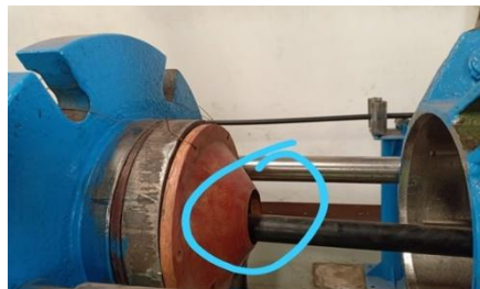
Figure 9. The part of the tube process that leak
