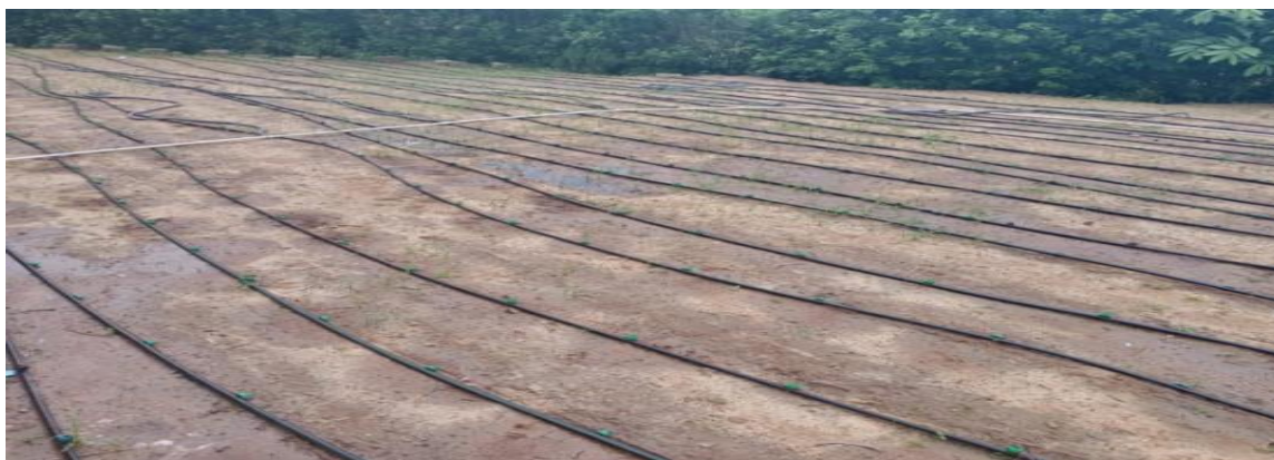
Fig: System At Sophitorium Campus
