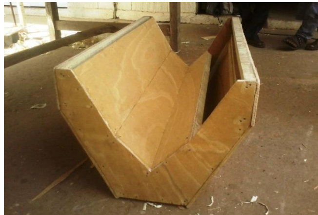
Figure 2.3: Assembling frame's top
