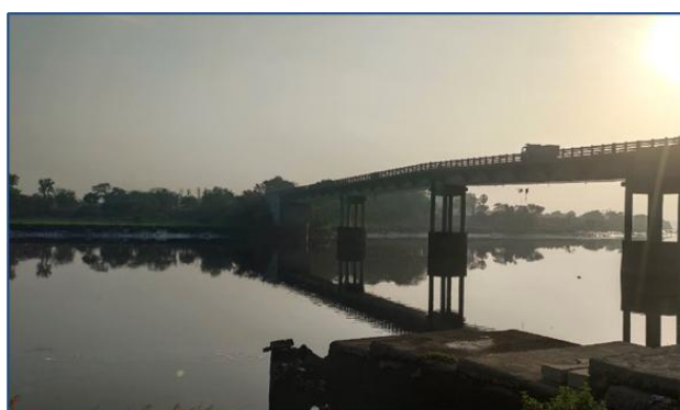
Fig.5: Survey area of the river near a bridge
