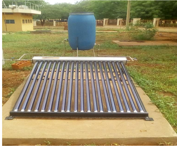
Plate 1: Evacuated tube collector type solar water heater
